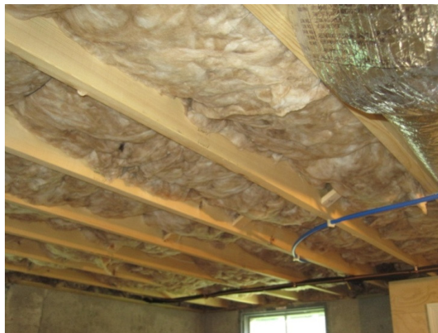
Figure B-13: Grade II Fiberglass Batts—Frame Floor
