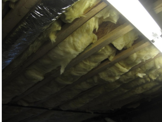
Figure B-14: Grade III Fiberglass Batts—Frame Floor
