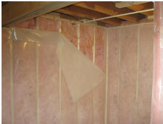
Figure B-11: Grade II Fiberglass Batts—Basement Walls
