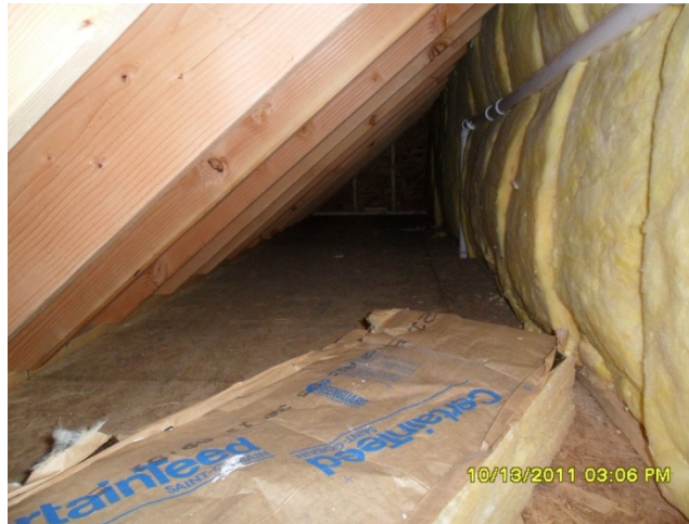
Figure B-12: Grade III Fiberglass Batts—Attic Kneewalls
